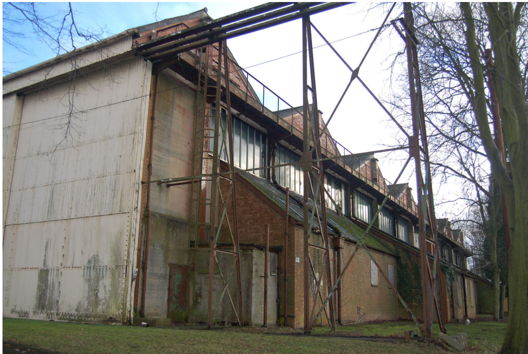
Building 79 A type hangar
